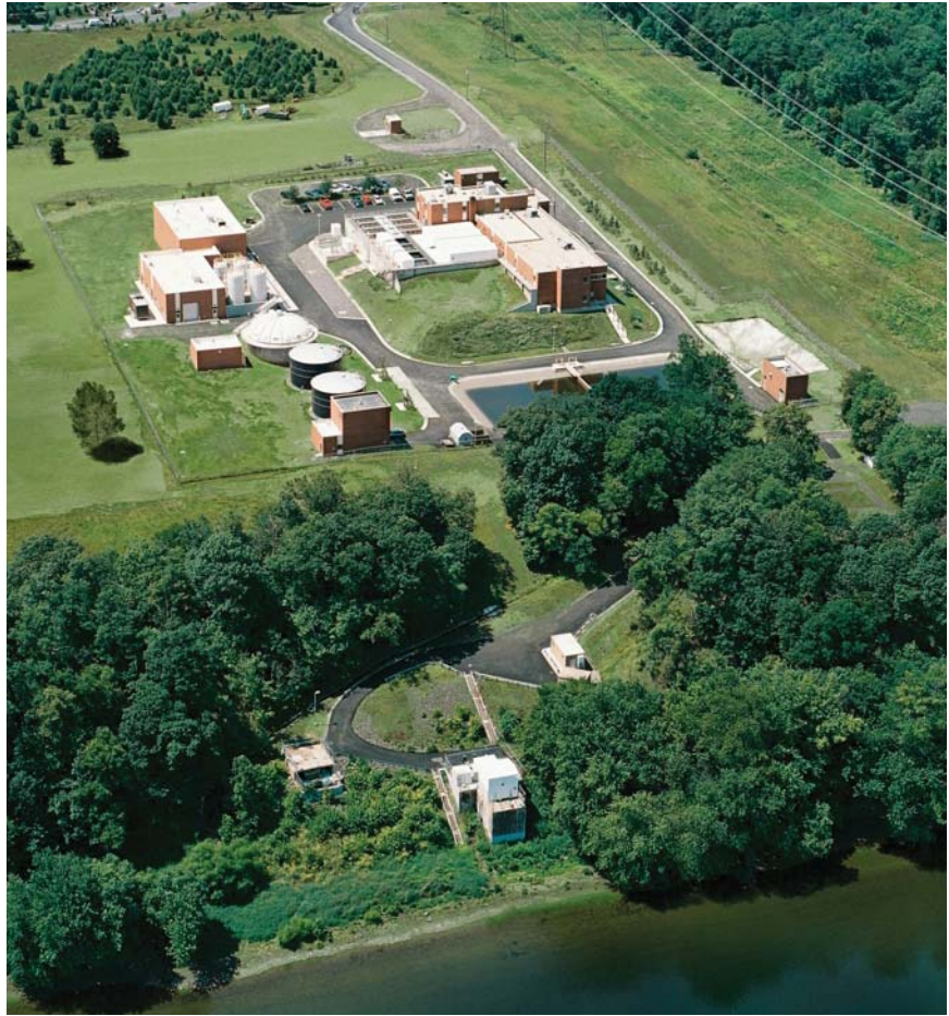
Fru-Con Construction seamlessly integrated new buildings and equipment into the existing facilities at the completed Kenneth B. Rollins Water Filtration Plant in Leesburg, Virginia.
