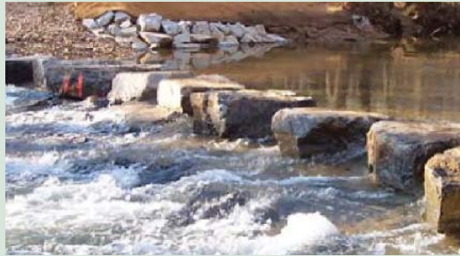
In Fairfax County, Virginia, Centennial restored the Difficult Run stream and added nature appreciation features.
