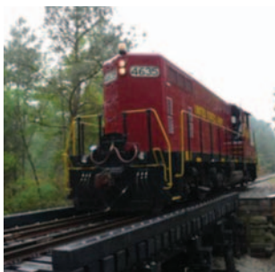
The U.S. Army's new recycled plastic railroad bridges require no substantial long-term maintenance.
