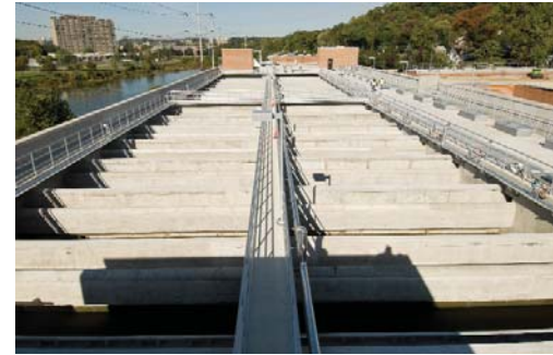
The 30,000-square-foot Filtration and Disinfection Facility at the Arlington plant rests on a 3.5-foot deep concrete foundation slab supported by 710 steel H-piles.
