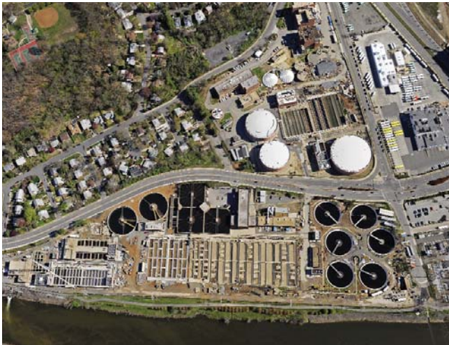
Fru-Con overcame a restricted 35-acre site to upgrade and expand the Arlington County Water Pollution Control Plant, surrounded by residential neighborhoods.
